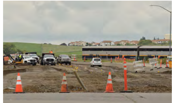
Jepson Parkway construction at Peabody Rd. and Vanden Rd., Fairfield
