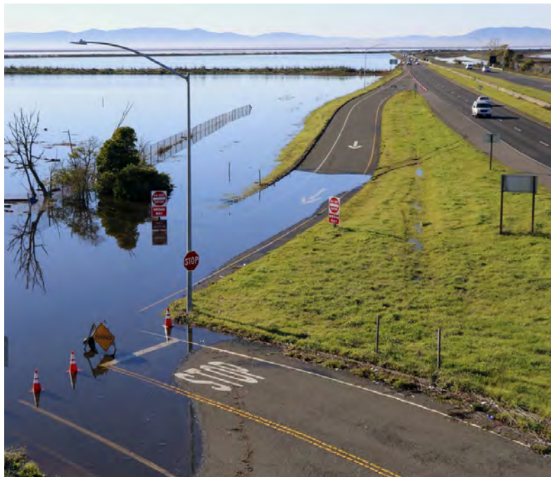
Flooding at SR 37/Walnut Ave offramp in Vallejo, March 2017
